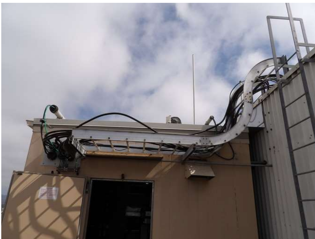
Antenna Cable Ice Bridge
