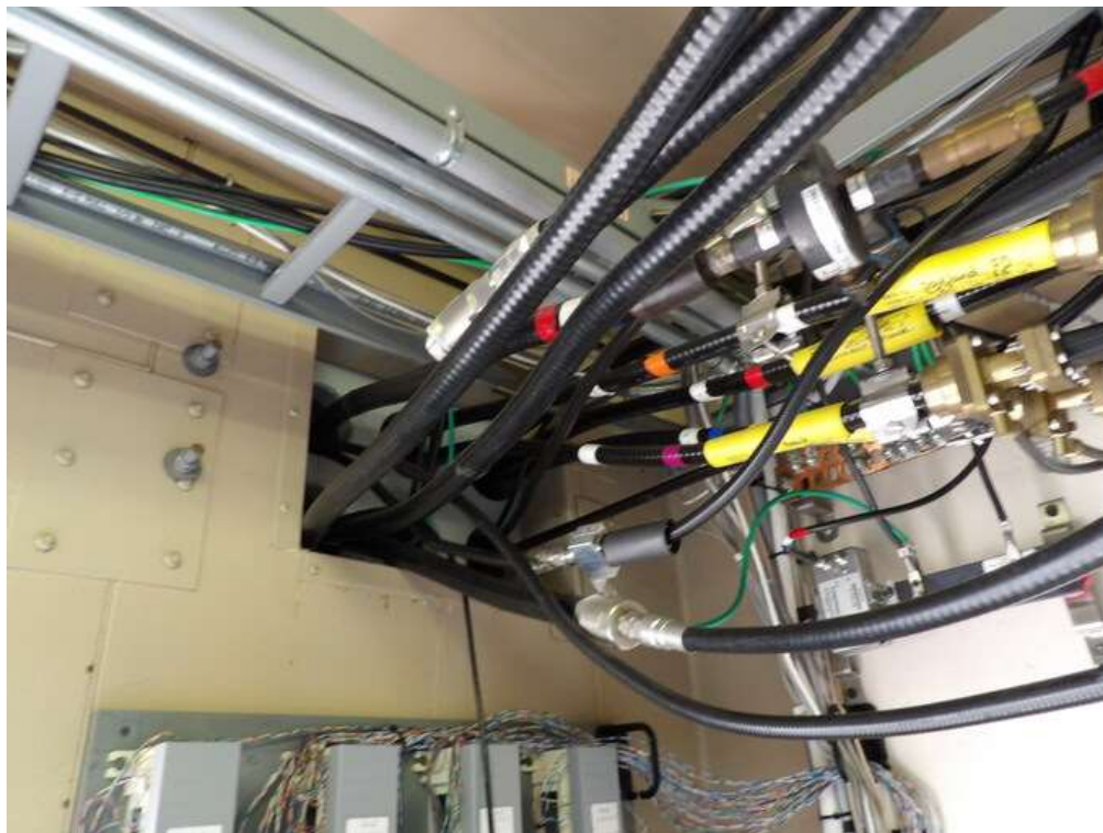
Antenna Interior Entry Port
