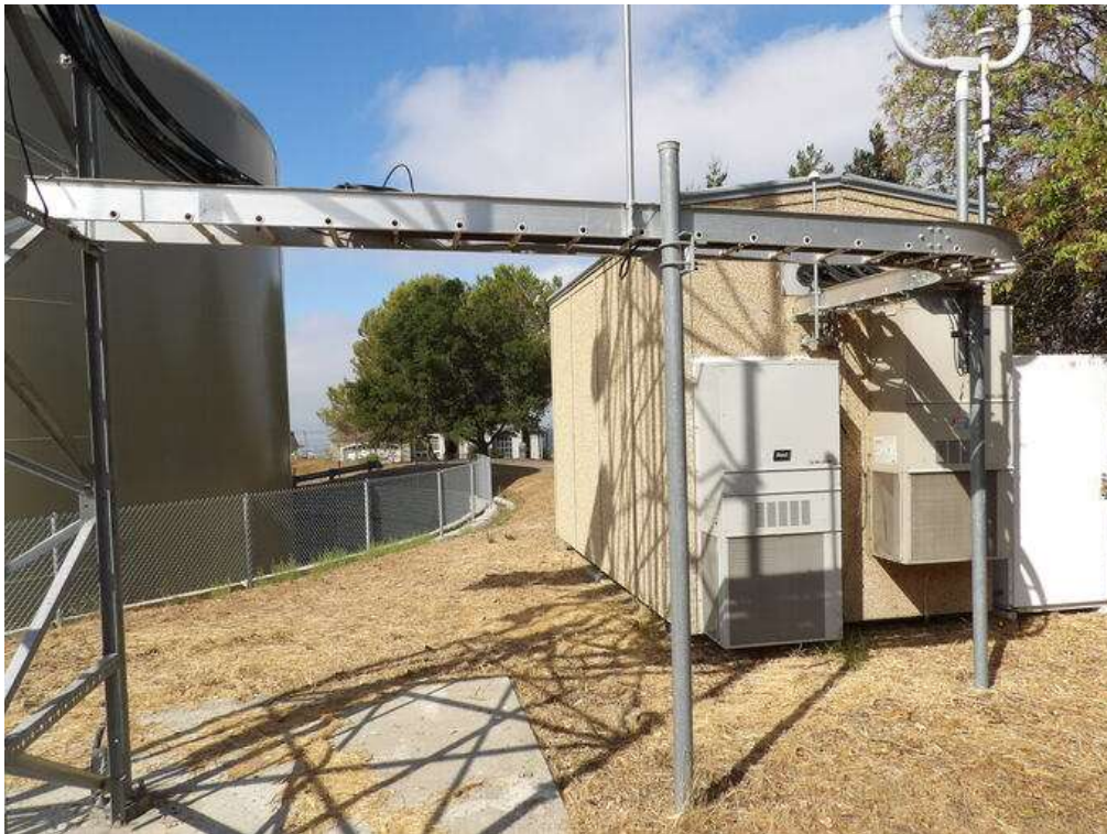
Antenna Cable Ice Bridge
