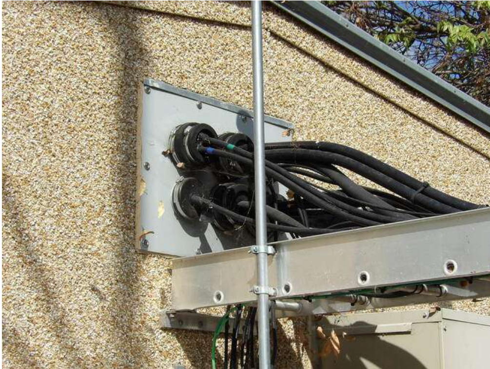
Antenna Exterior Entry Port
