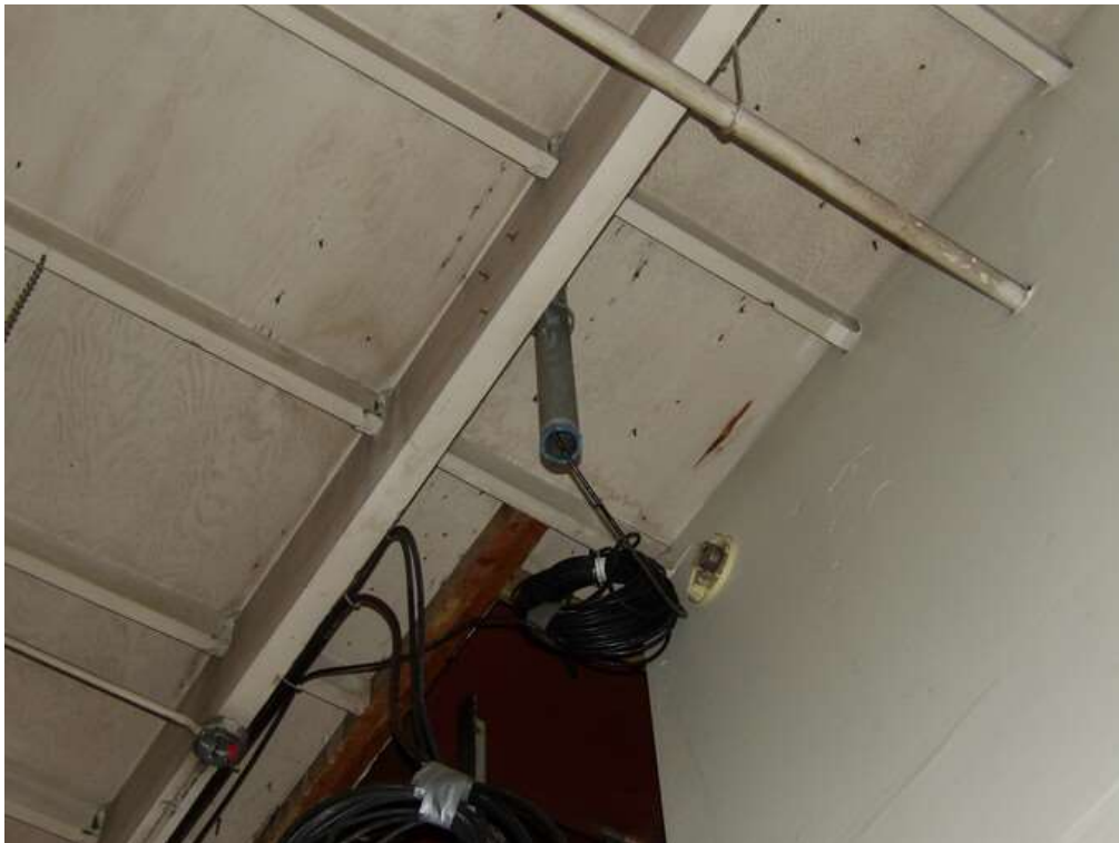
Antenna Cable Interior Entry Port
