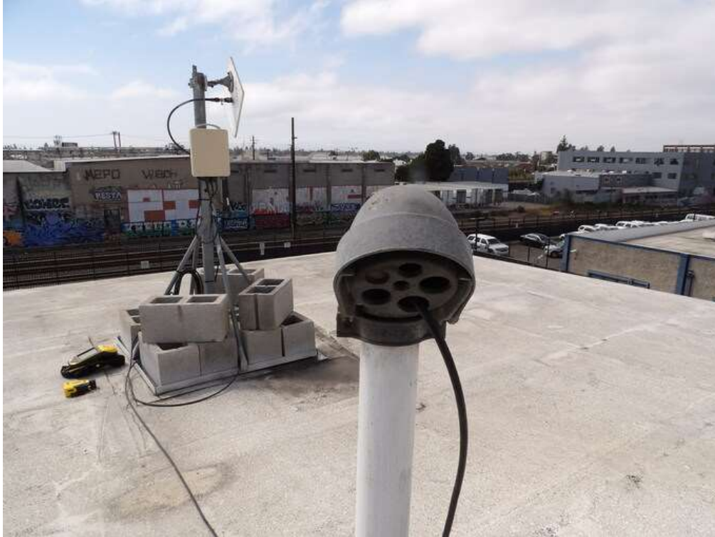
Antenna Cable Exterior Entry Port
