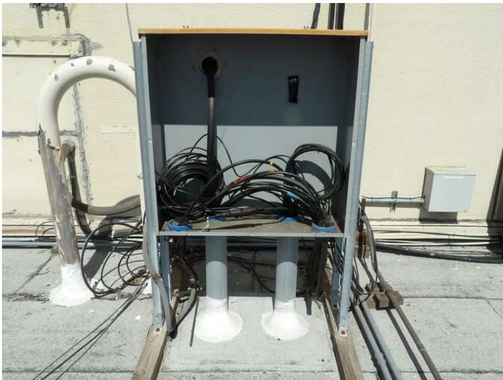
Antenna Exterior Entry Port
