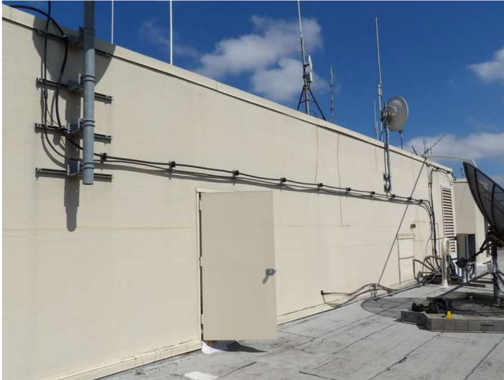
Antenna Cable Ice Bridge
