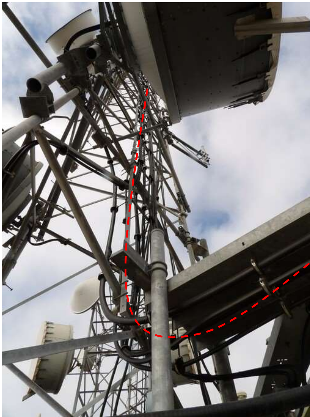
Antenna Waveguide Photo
