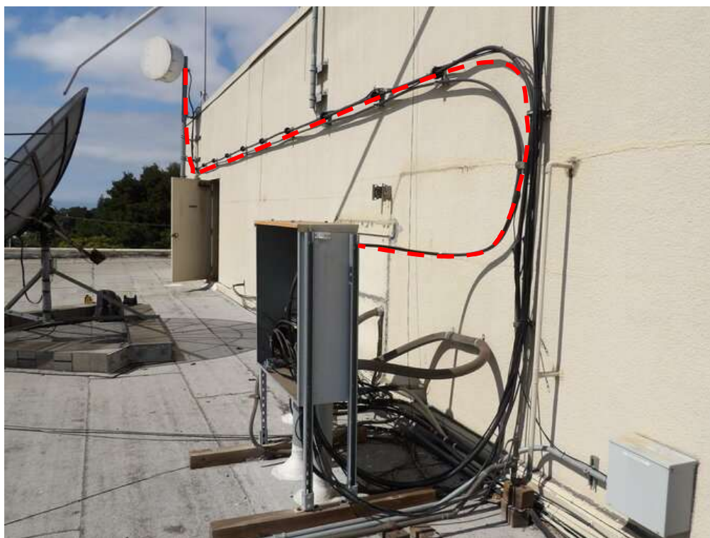
Antenna Waveguide Photo
